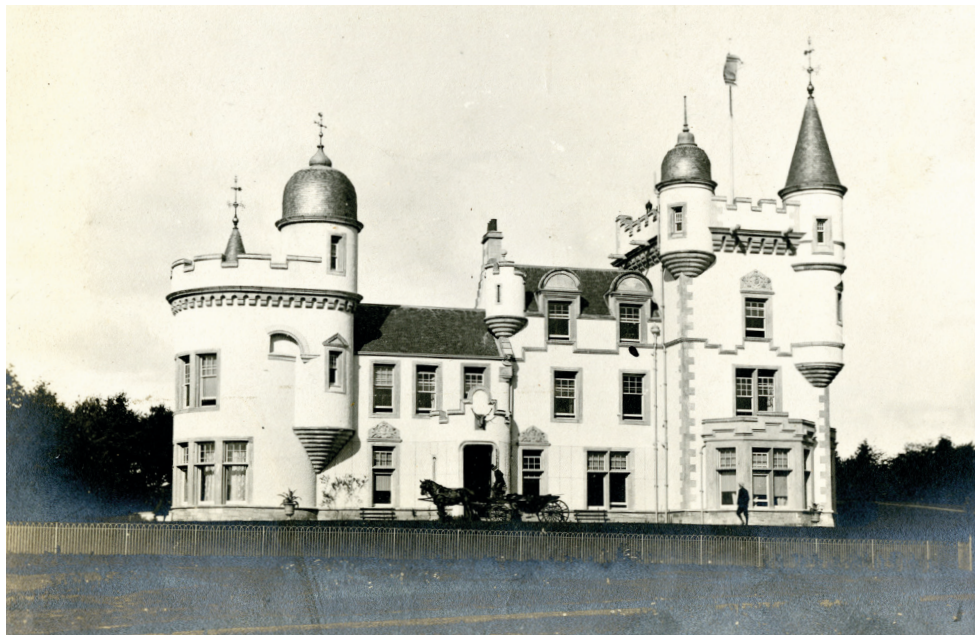
Feddal House, near Braco, c1905
