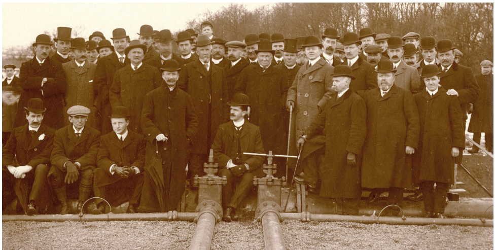
Crieff Waterworks Opening of Sewage Purification Works, 1909 Ref: CR/Papers/Bundle 10/Ph5
