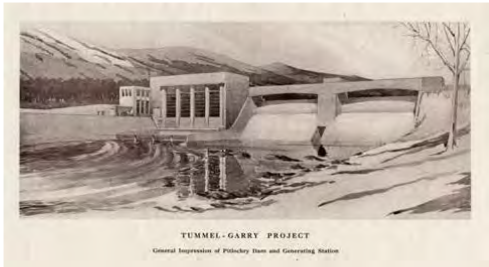
Below: Tummel Garry Project, Pitlochry Dam, c1945 Ref: PTC/427/1
